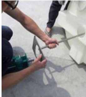
1. Put the tank down and install the pad
